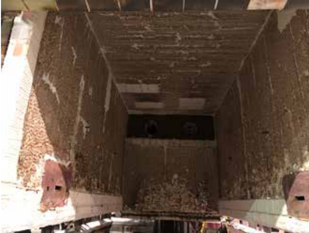
Forging furnace with old and badly devitrified ceramic fiber lining
